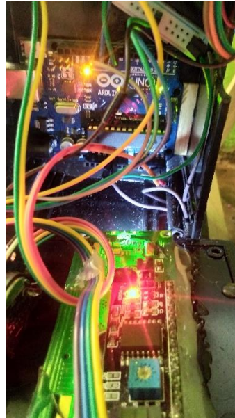
Figure 8. Power Supply Testing
